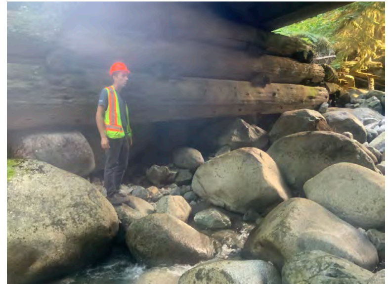
Right Bank Abutment when facing downstream
