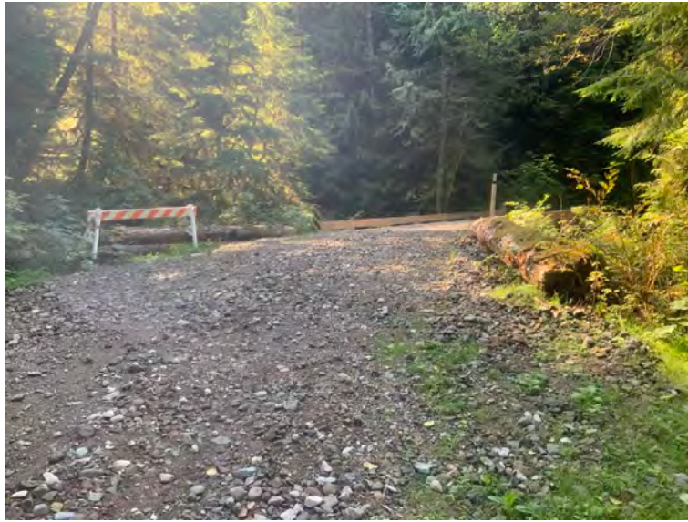
Approach from Right Bank when facing downstream
