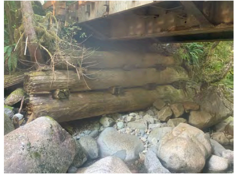
Left Bank Abutment when facing downstream
