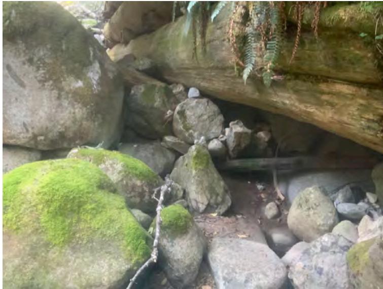
Left Bank Abutment when facing downstream
