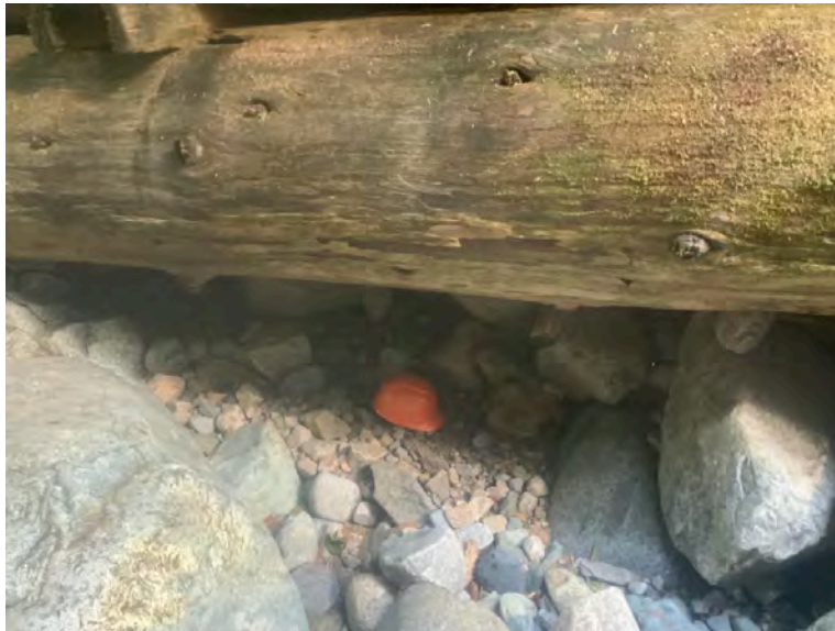
Right Bank Abutment when facing downstream
