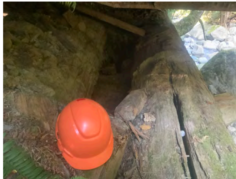
Left bank crib
