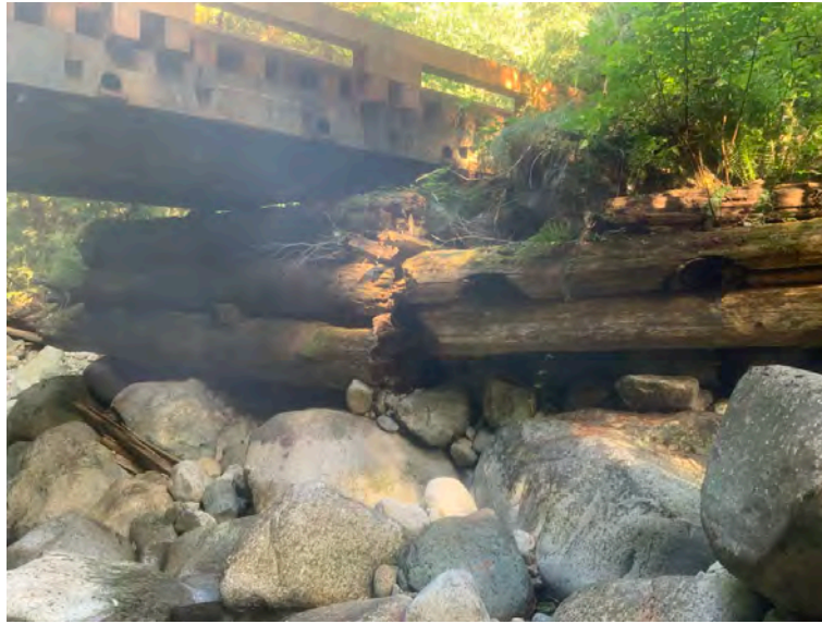
Right Bank Abutment when facing downstream
