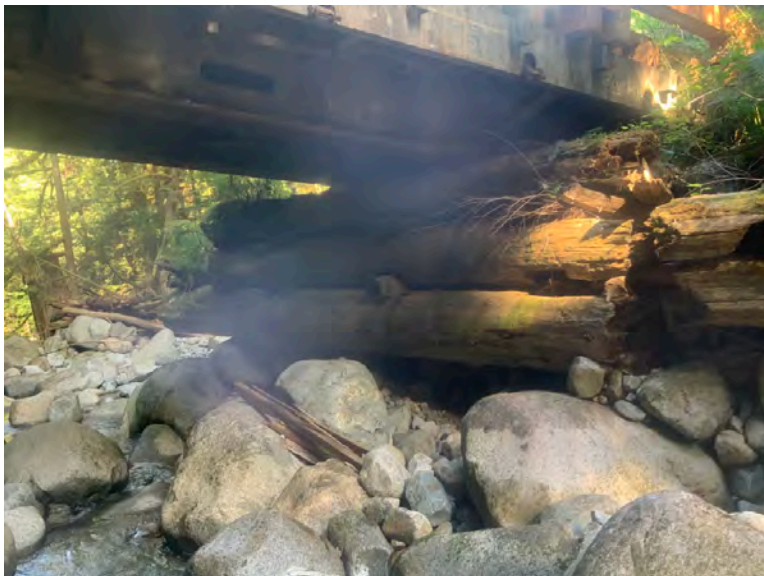
Right Bank Abutment when facing downstream
